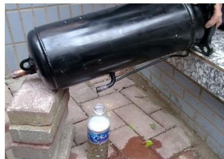
Figure 6-2.5: Draining oil from a compressor
